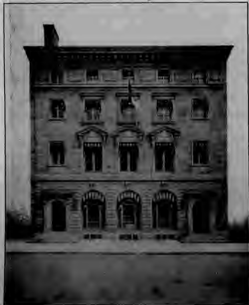
FIFTY-EIGHTH STREET BRANCH, Nos. 121 to 127 East Fifty-eighth Street, Borough of Manhattan.
